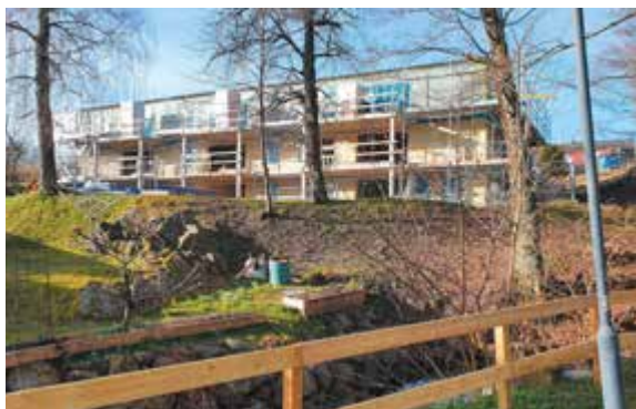
Blue wall Construction AB, Jönköping
