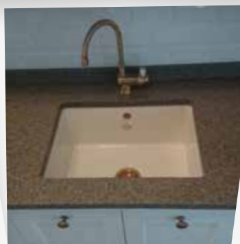
Installation i kök
